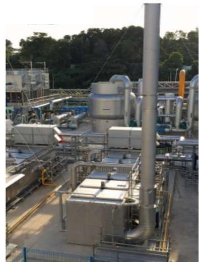
The vaporizer design can offer heat transfer efficiencies in the tube bundle and providing highly efficient regasification for cryogenic or refrigerated gases fluid such as LNG, Liquid Nitrogen, Liquid Oxygen, Propane, Ethylene and Butane.
